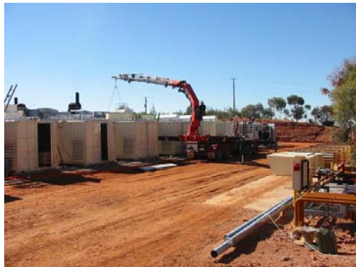
New Power Station under construction
