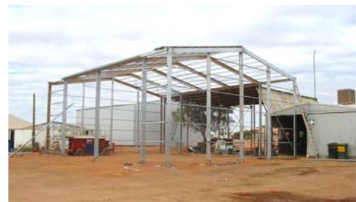
New Distribution Shed under construction
