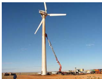
Cleaning the wind turbine tower
