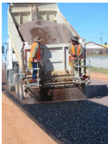
Road Sealing in progress
