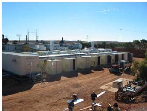
New Power Station under construction
